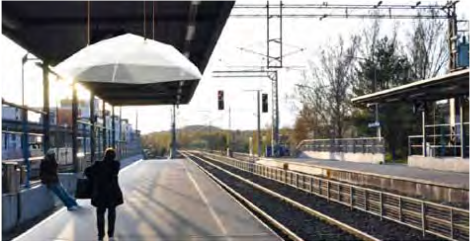
A protective canopy in the train station.
